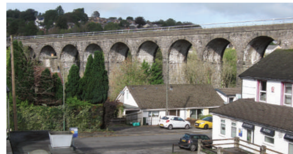
HENGOED VIADUCT: The former rail line is now used for a cycle path Picture: Julian Langston
