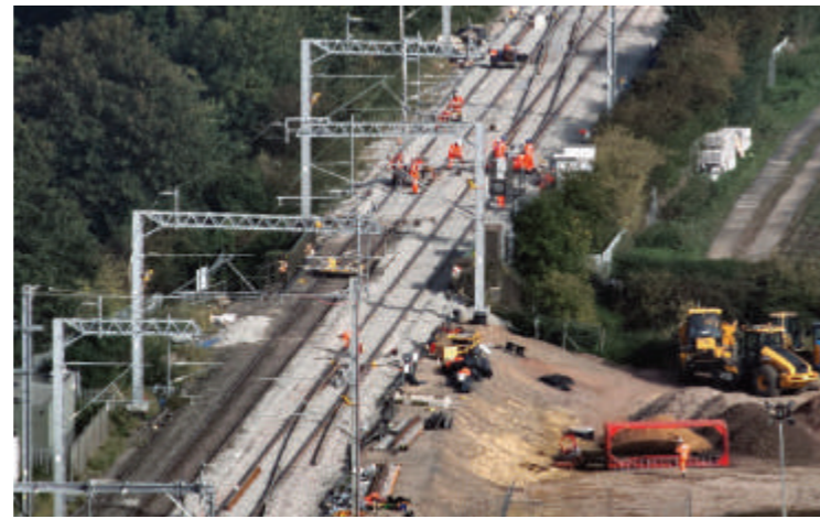
Aerial view of work to connect to main line
