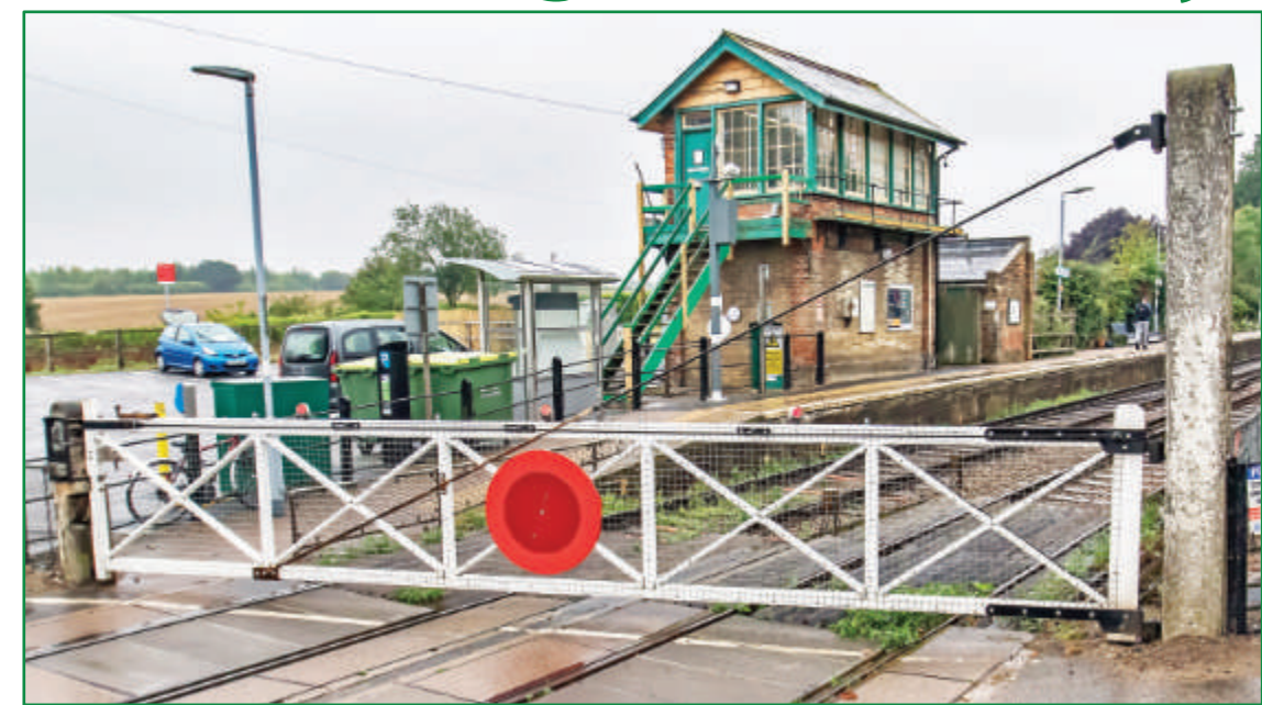
An increasingly unusual sight: Full-width staff-operated crossing gates. Dullingham in August 2021
