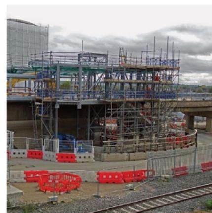
**Work on the new East West Rail station at Bletchley was making good progress in November. This view from Brunel roundabout on the east side of the line shows that the station will have a new, bold “face” towards the town centre. Work has involved demolishing sections of the 1960s flyover to make a secure bridge over the West Coast main line and to create space for the new station entrance**
