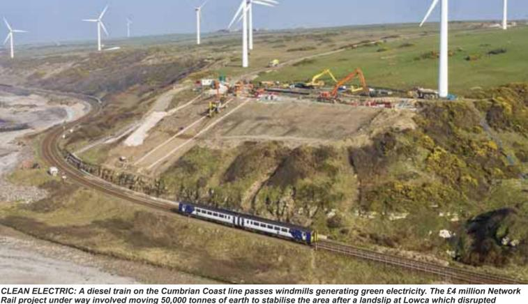
Rail project under way involved moving 50,000 tonnes of earth to stabilise the area after a landslip at Lowca which disrupted passenger and freight trains running between Carlisle and Whitehaven
