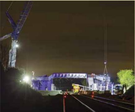
HORDEN: A 500-tonne crane was used to position the footbridge deck, stairs and ramps in April for the station between Hartlepool and Sunderland
