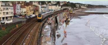
Network Rail has installed a bigger sea wall at Dawlish, Devon, to protect the coastal line following the repeated breaches by the sea over the past few years. The line connects 50 towns and cities in Devon and Cornwall with the rest of the country. Railfuture believes the line between Dawlish and Teignmouth is so vulnerable that an alternative route should also be made available by reopening the line via Okehampton.
