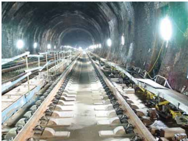
CONTRAST: New track and Victorian brickwork in the tunnel
