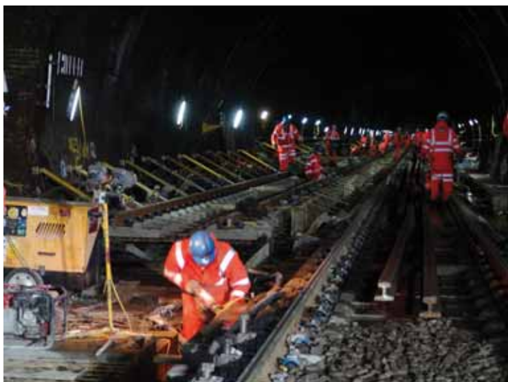
TEAMWORK: Southampton tunnel
