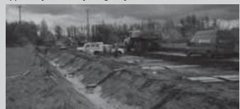
sections. Strange that this wasn't considered when the route was designed! Steve Wilkinson's pictures show how the process of wrecking a railway, above, and digging a four-foot ditch was continuing in May at Histon. Below: The concrete sections of the busway are put in place by a huge beam-laying machine. This is where two main lines and a mile-long goods loop used to be. What a waste!
