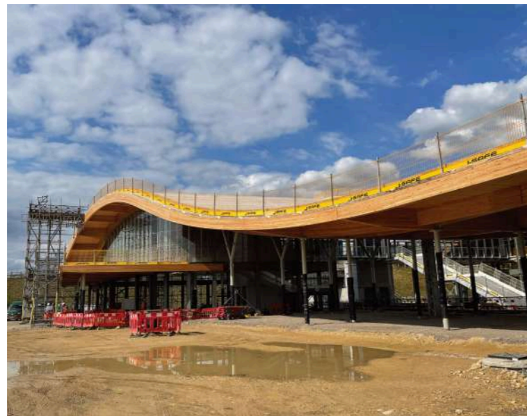
SWEEPING AHEAD: Cambridge South station during construction
