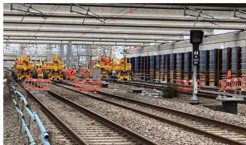
Picture: NETWORK RAIL
