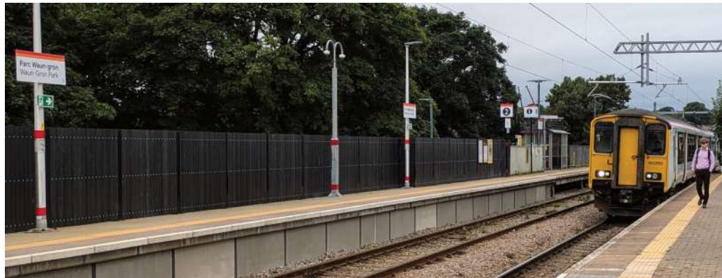
Major improvements for Cardiff Valley lines: Platform extensions at Waungron Park and new electrification Picture by Julian Langston
