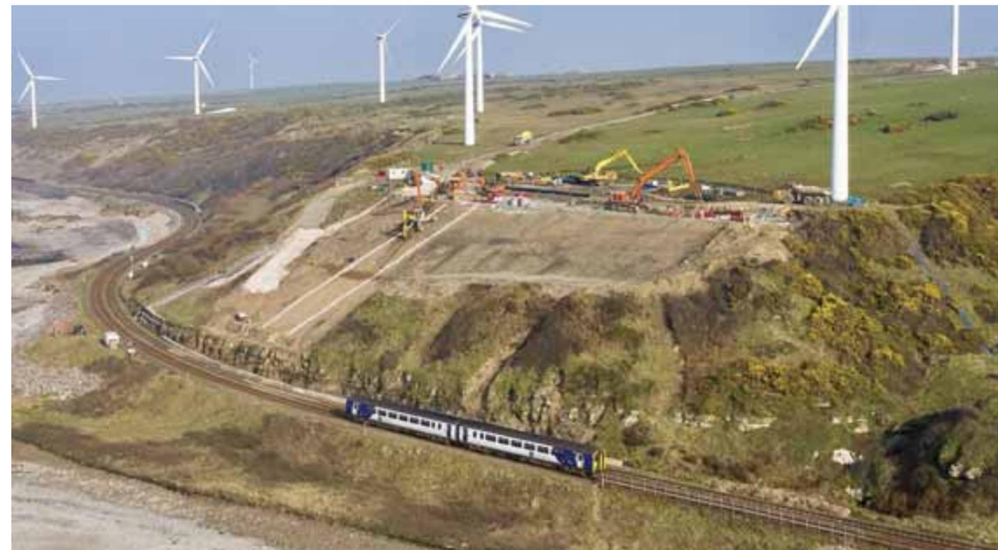
**CLEAN ELECTRIC:** A diesel train on the Cumbrian Coast line passes windmills generating green electricity. The £4 million Network Rail project under way involved moving 50,000 tonnes of earth to stabilise the area after a landslide at Lowca which disrupted passenger and freight trains running between Carlisle and Whitehaven
