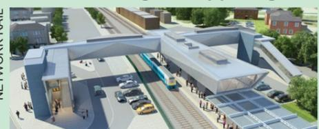
The new bridge at Port Talbot Parkway, pictured above, which includes a new ticket office, waiting areas and information points, as well as steps and lift access to all platforms, has been completed. Similar work at Llandaf and Radyr is well advanced with lifts and tactile paving. Work has started on a new bridge with slope for
