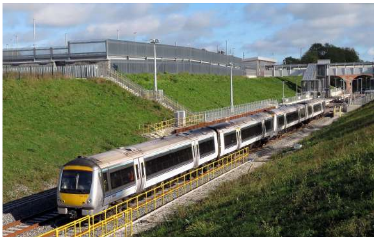
HIGH HOPES FOR EWR: Two Chiltern Railways class 168 diesel units pass the new Winslow station in October 2024. On the same day, a Great Western class 800 inter-city train also went through Winslow on a test run. Nearly two years later, no regular passenger trains have run
