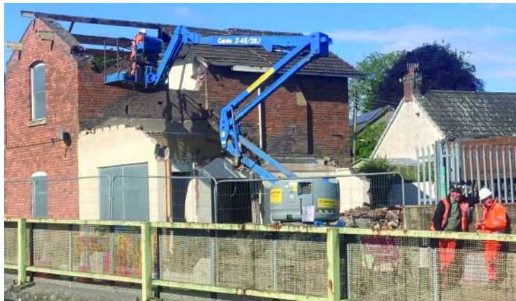
More than just a spade in the ground: Workers on the Portishead rebuilding project use an articulated boom lift to dismantle the old station house, reclaiming the bricks for further use and making way for work to start on Portishead's new station
