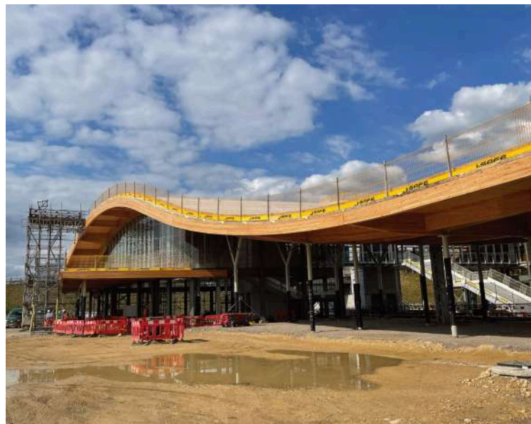
SWEEPING AHEAD: Cambridge South station during construction
