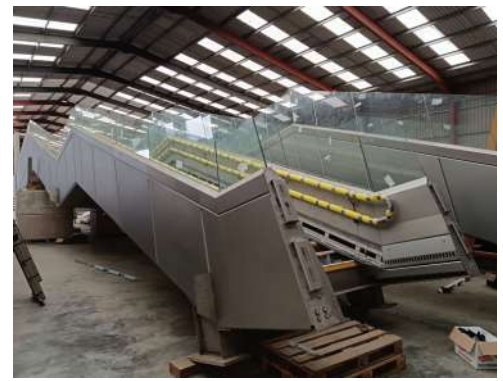
Prefabricated parts of the modular AVA footbridge before installation at Stowmarket station at the end of November
