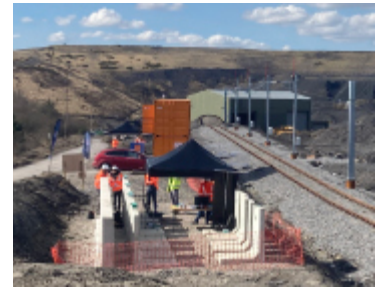
Mimicrete (foreground) and CODES (rear) test areas
