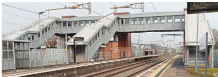
Theale station's new, accessible footbridge
