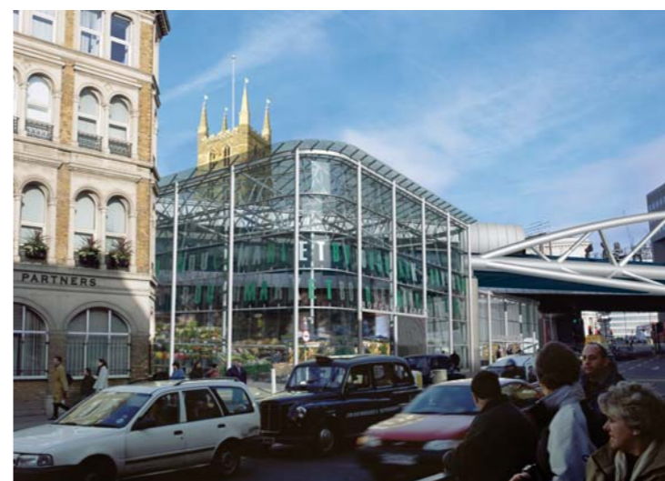
THAMESLINK: Work has already started in London on the Borough Market viaduct for the Thameslink scheme
