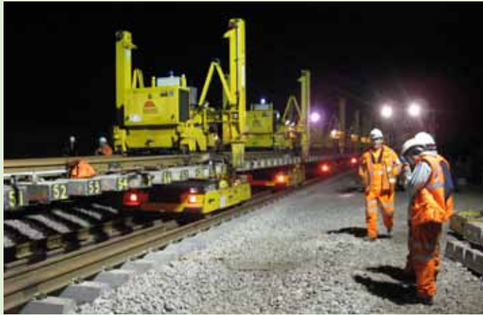
Picture: NETWORK RAIL
