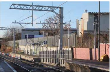
SPOT THE DIFFERENCE: Tram-train operation through main line stations is liable to involve the provision of lower platforms to match the lower platforms on the tramway. The difference is shown in this view of the Parkgate-bound tram-train platform at Rotherham Central (platform 4) compared with the main line platform 2 to the right.
