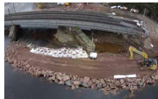
**DAM:** Engineers built a temporary dam in January round two piers of Lamington viaduct on the West Coast main line in Scotland after the line was undermined by floods. The line through Lamington was closed for seven weeks
