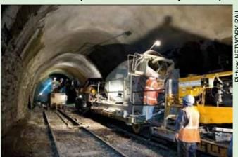
Cement spraying to strengthen Whiteball tunnel
