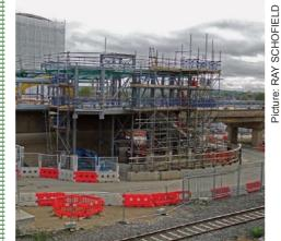
Work on the new East West Rail station at Bletchley was making good progress in November. This view from Brunel roundabout on the east side of the line shows that the station will have a new. bold "face" towards the town centre. Work has involved demolishing sections of the 1960s flyover to make a secure bridge over the West Coast main line and to create space for the new station entrance
