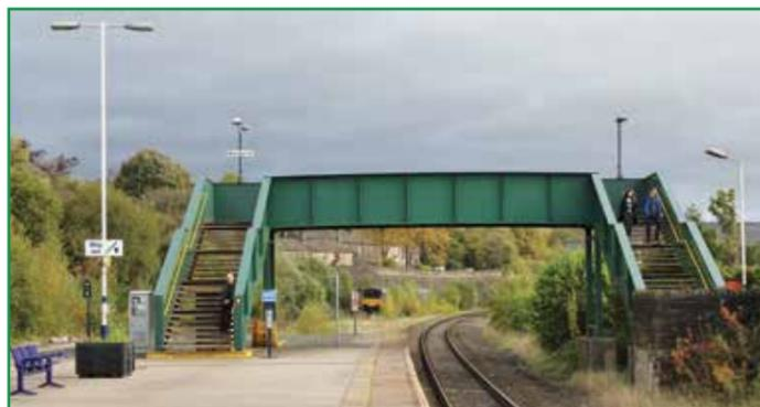
**FOOTBRIDGE AS BARRIER:** Trains at Chinley station call at either side of this island platform, which can be reached only by the green footbridge. The 24 steps visible on the left are matched by a similar number on the right. The whole bridge is open to the weather and tricky even for able-bodied passengers in the wet, especially if they have luggage or young children
