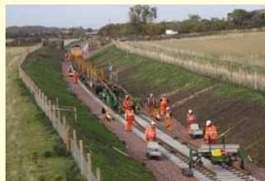
Work under way: An engineering train on freshly laid track and workers lay rails
